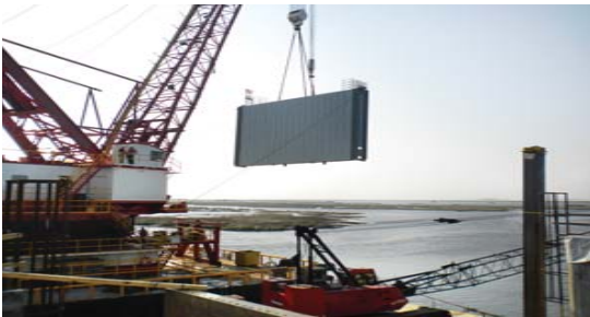
Example Installation of a Flood Gate
