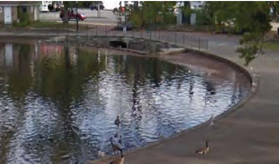
Existing Weir and Blocked Box Culvert at Halls Pond
