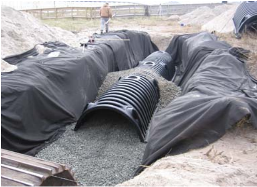
Construction of Subsurface Retention
