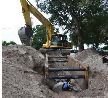
Example Replacing Drainage Pipe for Lawson Blvd.
